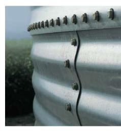
**Strong sidewall sheets** feature 4-inch (102-mm) corrugations. In addition, each BROCK<sup>®</sup> Sidewall Sheet is 44 inches (1118-mm) wide which reduces erection costs because the bin goes up faster.
